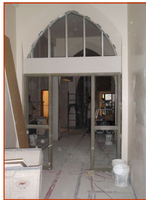
Second Floor remodel.
